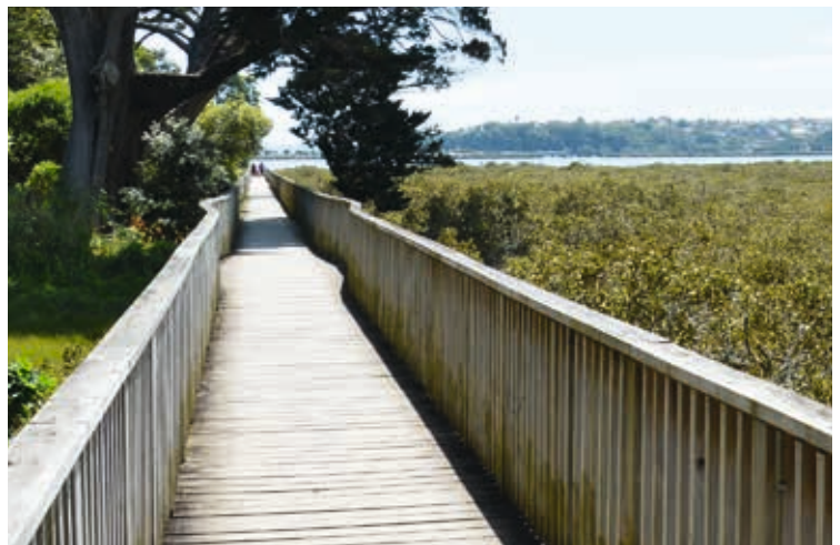
Pathways built by the Orakei Local Board around inner Hobson Bay have the more aesthetically harmonious timber balustrading. Photos: Stephen Penny
